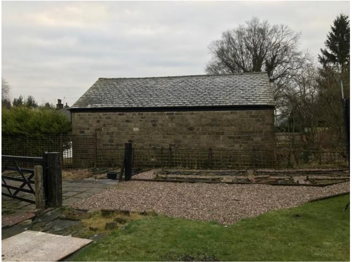
Garden - overlooked by skylights and large glazing in extensions
